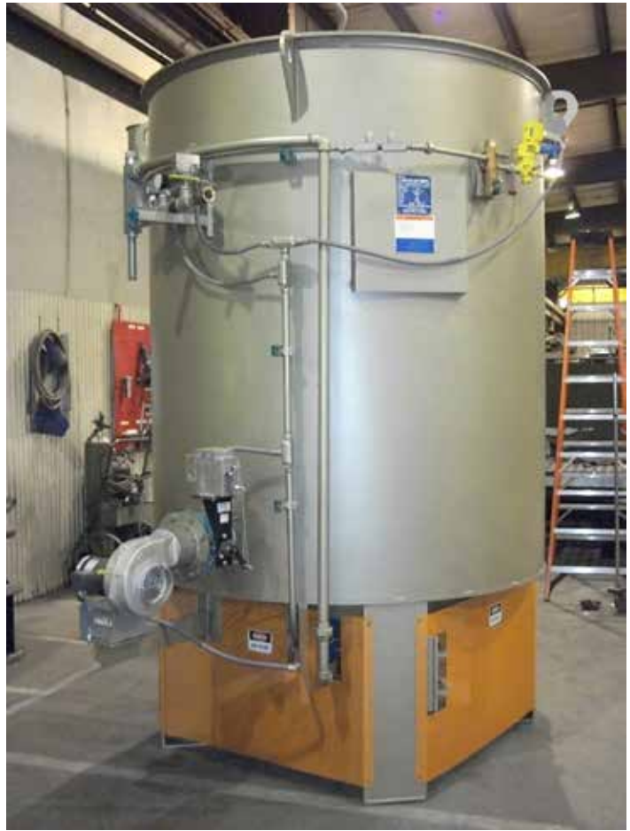
Figure 2: Steam treating with cooling blower.
